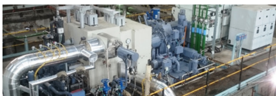
Following the removal of older turbines, three turbines being installed at Saiccor and Tugela Mills will increase our net generating capacity by 23MW, making us less dependent on the national grid, reducing costs and insulating us from electricity price increases from FY17 onwards. Tugela Mill's turbine shown.
